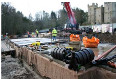
With the basement complete, work begins on the ground floor. December 2008
